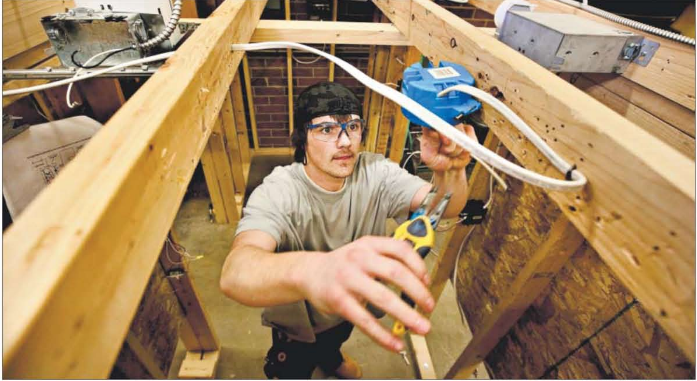
Michael MacNeil, 18, who is a student at Warren Tech, learns how to wire a light fixture Thursday at Red Rocks Community College in Lakewood. LINDA MCCONNELL/SPECIAL TO THE ROCKY
